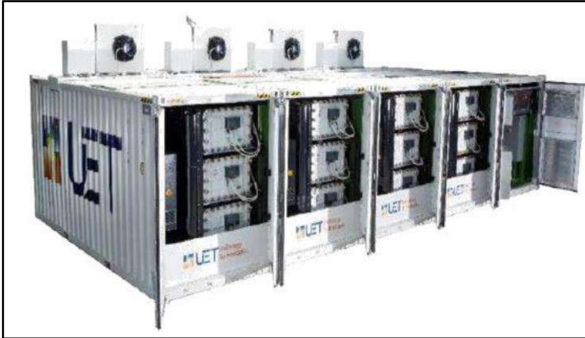
**Figure 10: Flow Batteries - Vanadium Redox Battery**
